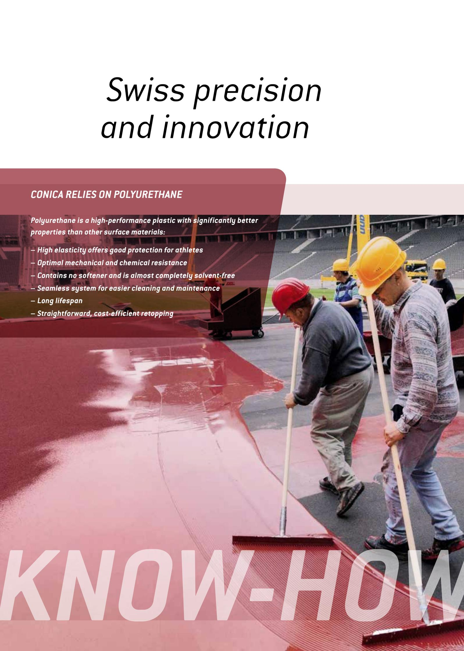
A photograph showing construction workers in hard hats and work clothes applying a red polyurethane coating to a large, flat surface, likely a stadium floor. The workers are using long-handled rollers. The background shows stadium seating and construction equipment.
