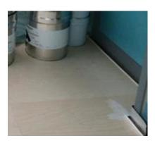
The application of CONIPUR 3330 (CONIPUR 227) is done with a notched squeegee. The consumption is approximately 2.2 kg/m $^2$  (2.8 kg/m $^2$ ) to obtain a 2 mm layer.
